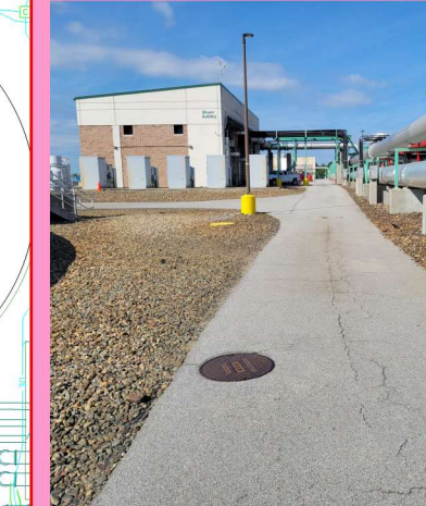
MILL AND REPLACE TO MATCH THE NEW PAVEMENT TO EXISTING MANHOLE ELEVATION.
