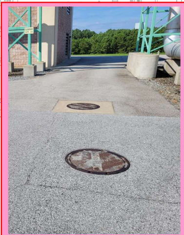
MILL AND REPLACE TO MATCH THE NEW PAVEMENT TO EXISTING MANHOLE ELEVATION.
