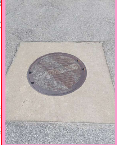
MILL AROUND CONCRETE COLLAR WITHOUT DISTURBING. SAWCUT BROKEN EDGE OF CONCRETE AND REPLACE.
