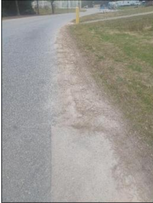
Photo 5: View of pavement edge near scale
