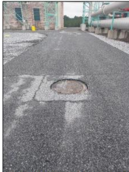
Photo 4: View of Depressed MH Cover Collar
