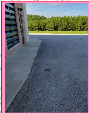
ADJUST WATER VALVE BOX TOP TO MATCH NEW PAVEMENT ELEVATION WITH A RISER RING AS MANUFACTURED BY EJ COMPANY.
