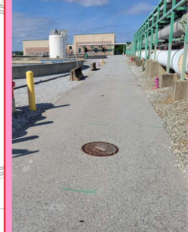
MILL AND REPLACE TO MATCH THE NEW PAVEMENT TO EXISTING MANHOLE ELEVATION.
